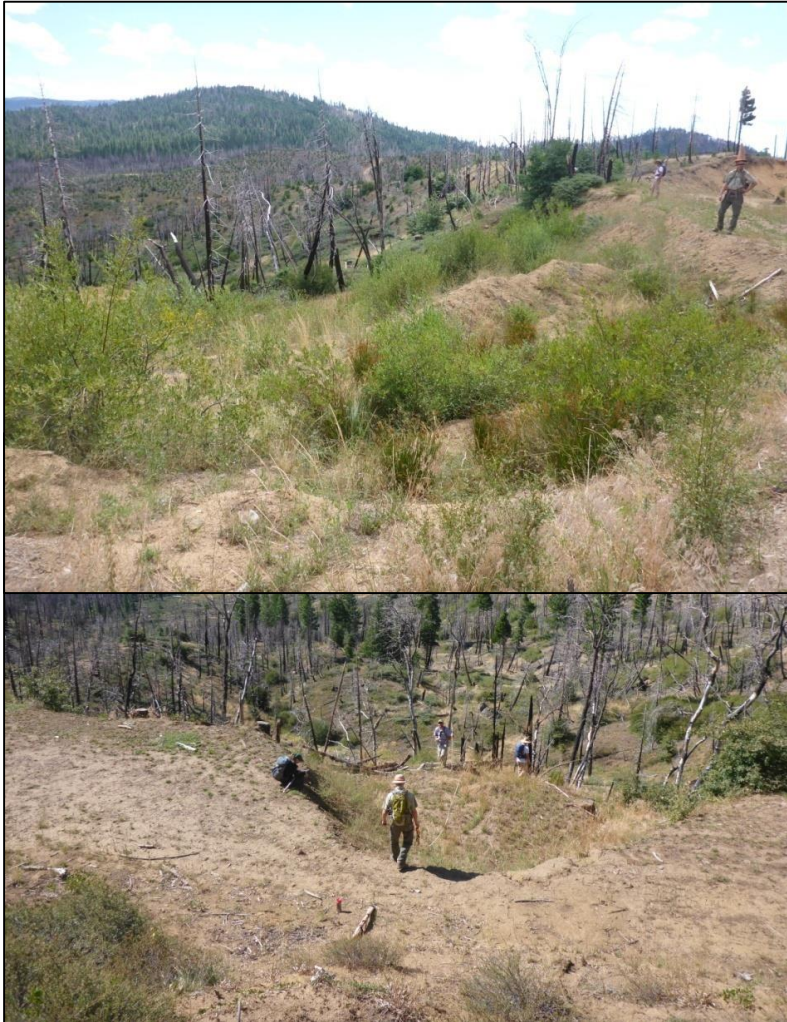
Figure 19. Fillslope failure type landslides in earthflow terrain.
