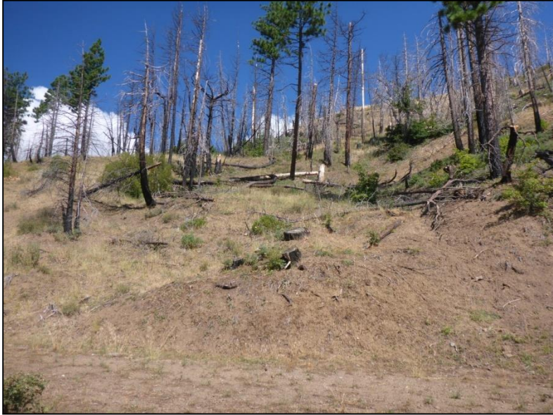
Figure 18. Cutslope failure type landslide in earthflow terrain.
