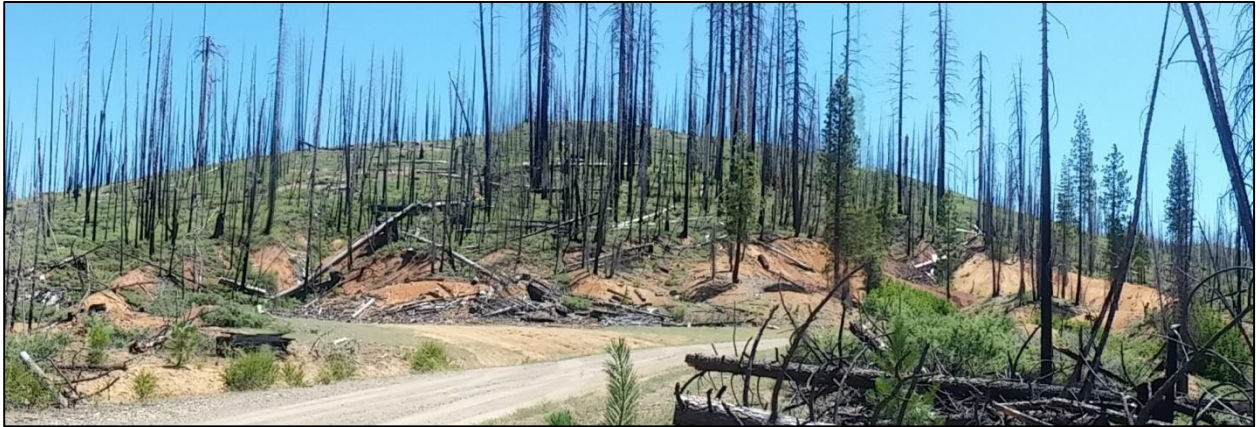
Figure 2. Photo showing red oxidized soil with lack of vegetation from severe burn intensity on old mining features along 28N30 in West Lights Creek.
